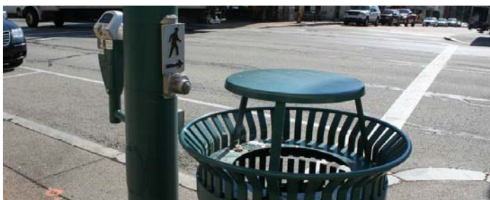
Obstructed, non-ADA compliant push button (Washington Rd. at Central Sq.)
