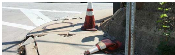
Damaged sidewalk, non-ADA compliant pedestrian sidewalk and ramp (McFarland Rd. at Washington Rd.)
