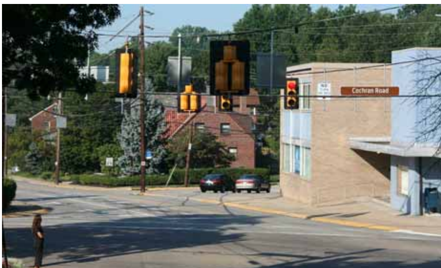
Figure 10 – Obstructed Traffic Signals and Mountable Curb (Cedar Boulevard at Cochran Road)
