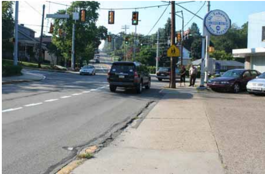
Figure 8 – Lack of Defined Sidewalk at Driveway Crossings (Cochran Road at Cedar Boulevard)
