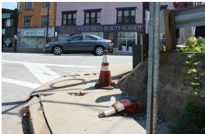
Figure 7 – Damaged Sidewalk, Non-ADA Compliant Pedestrian Sidewalk & Ramp (McFarland Road at Washington Road)
