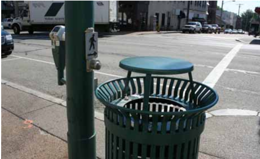
Figure 5 – Obstructed, Non-ADA Compliant Push Button (Washington Road at Central Square)
