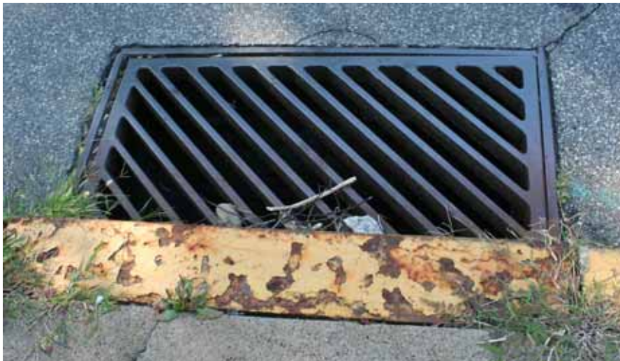
Figure 9 – Non-Bicycle Safe Grate (Cedar Boulevard at Cochran Road)
