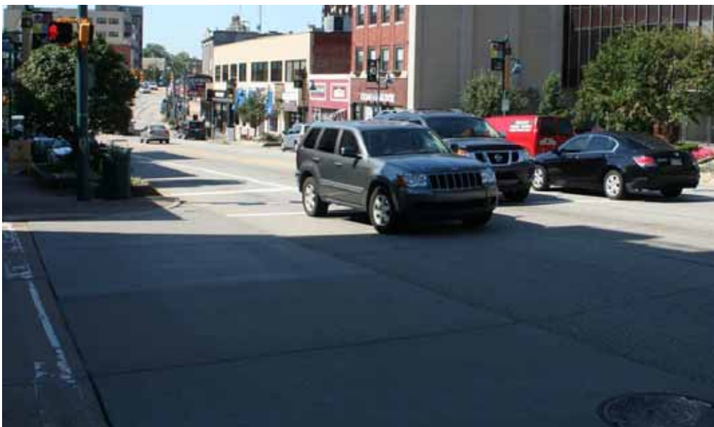
Figure 4 – Crosswalk Markings not Visible (Washington Road at Cedar Boulevard)
