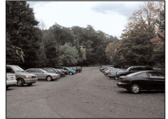
Parking lots, such as this one along Beadling Road in Bird Park, can be rebuilt to actually cleanse storm water run-off.
