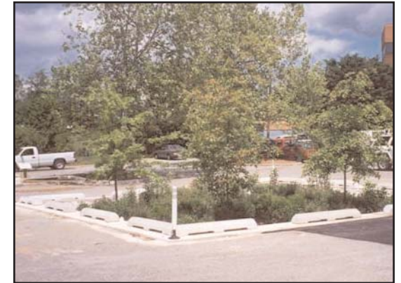
This is one example of a storm water cleansing parking lot. Rain water is directed towards this central island, where it is cleaned before being released (photograph courtesy of Biohabitats, Inc.).
