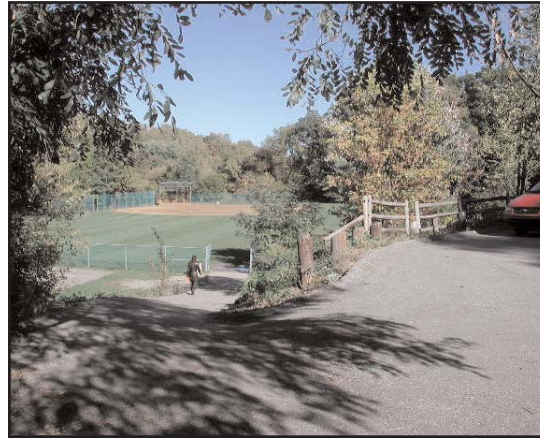
Entry is poorly defined and blends into street paving. Slopes and entrance walkway are very steep.
