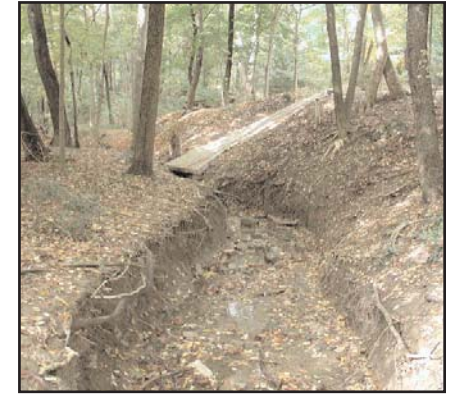
Severe erosion causes topsoil to wash away, exposes roots and threatens the stability of the adjacent stream banks.
