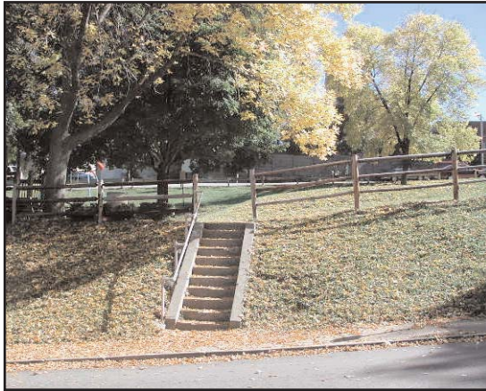
Grass on the slope between Lavina Avenue and the park should be removed and the bank stabilized with a low-maintenance groundcover. Additional steps will provide more ways to get up to the park.
